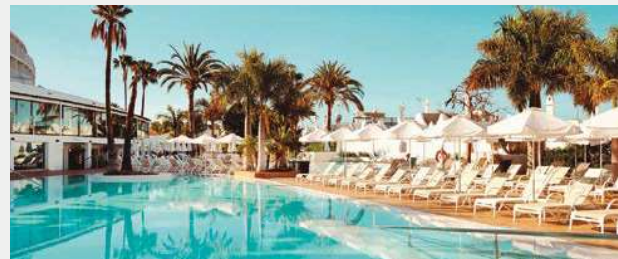
Thomas Cook's Sunprime Atlantic View resort. A holiday resort in the Canaries. Spain. 229 rooms plus full spa and swimming pool facility.
